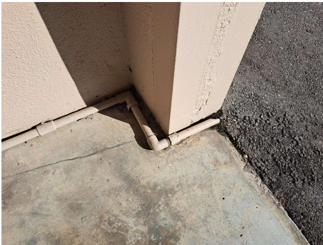
Photo 01 Ref: 2.1.1.1 – Air Conditioner Draining Next To Foundation
